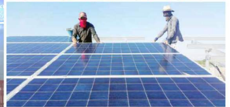
Technical staff install solar panels.
